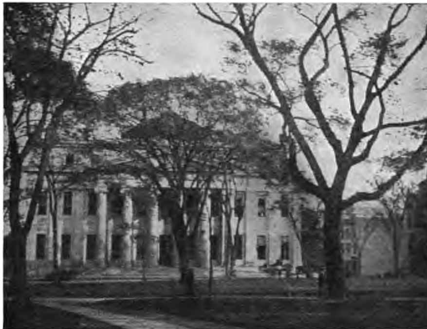
City Hall, Albany, N. Y. A good example of a public building with adequate open space to give it a proper setting
